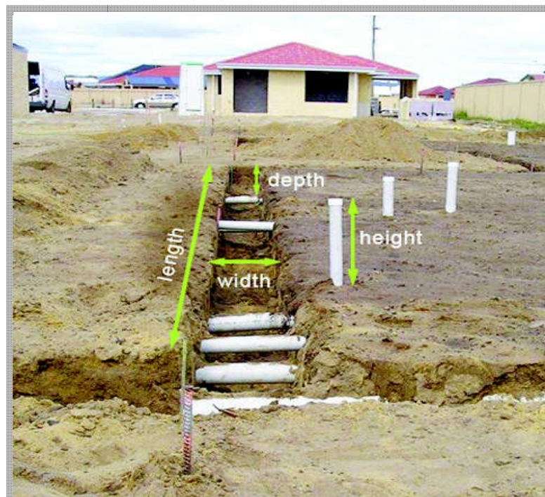
Figure 2.3 trench excavation
